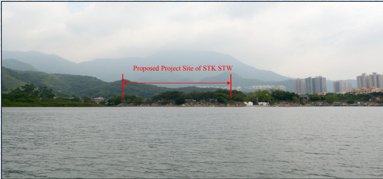
View of VSR - T2:
