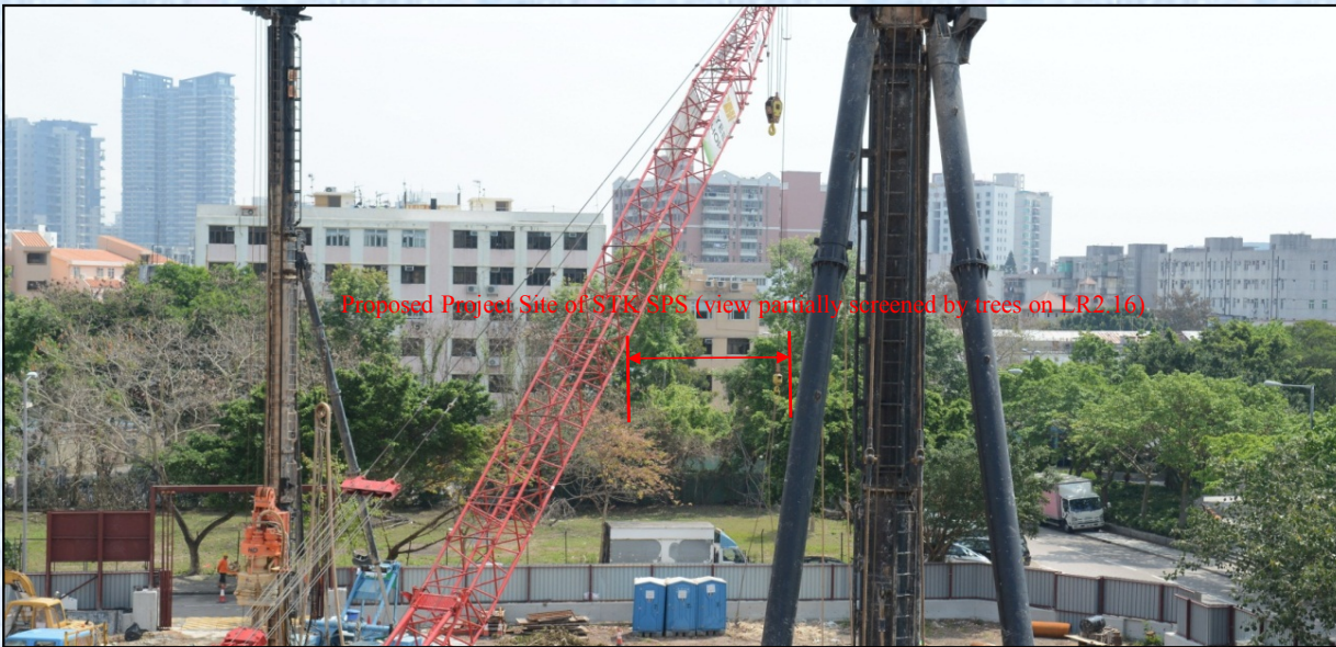
View of VSR - R6:
