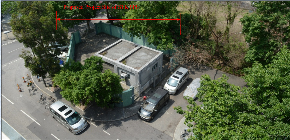
View of VSR - R5:
